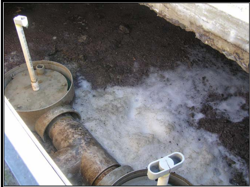
19 th June 2007: Day 1 of aeration and bacteria dosing. Surface crust 20cm thick
