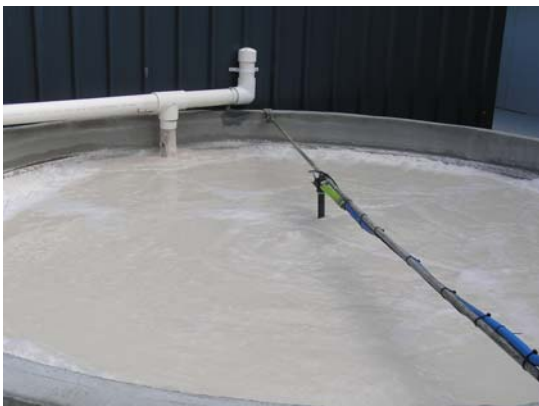
Aeration and dosing of tank
