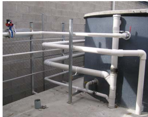
Top water allowed to settle and decanted for irrigation
